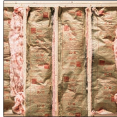
R-13 Batten Insulation In Walls & Ceiling
