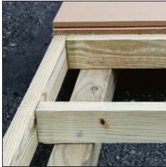
Pressure Treated 2x4 Floor Joists 4x6 Runners
